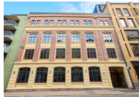
Calmeyers gate 12, Oslo 1 926 m 2
