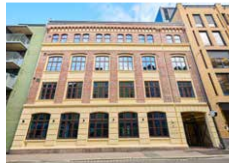
Calmeyers gate 12, Oslo 1 926 m 2
