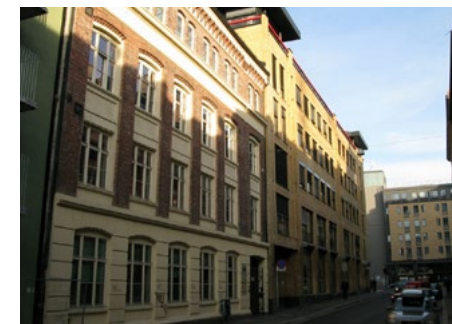
Calmeyers gate 12, Oslo
